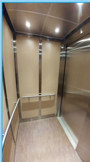
An elevator cab upgrade is optional when an elevator is modernized. The upgrade reuses the existing car and platform and sets new wall panels on the supporting shell structure that are separated with stainless steel reveals. As well, the face of the car and the front transom are capped in stainless steel and the hand railings are replaced to suit the current Code.
